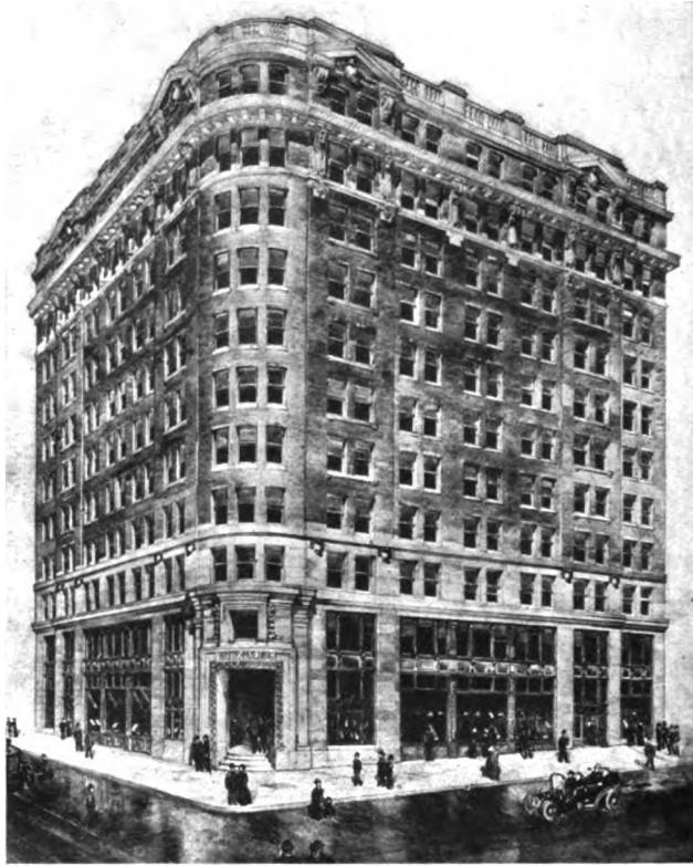
The White Building—Home of the Metropolitan Bank.
